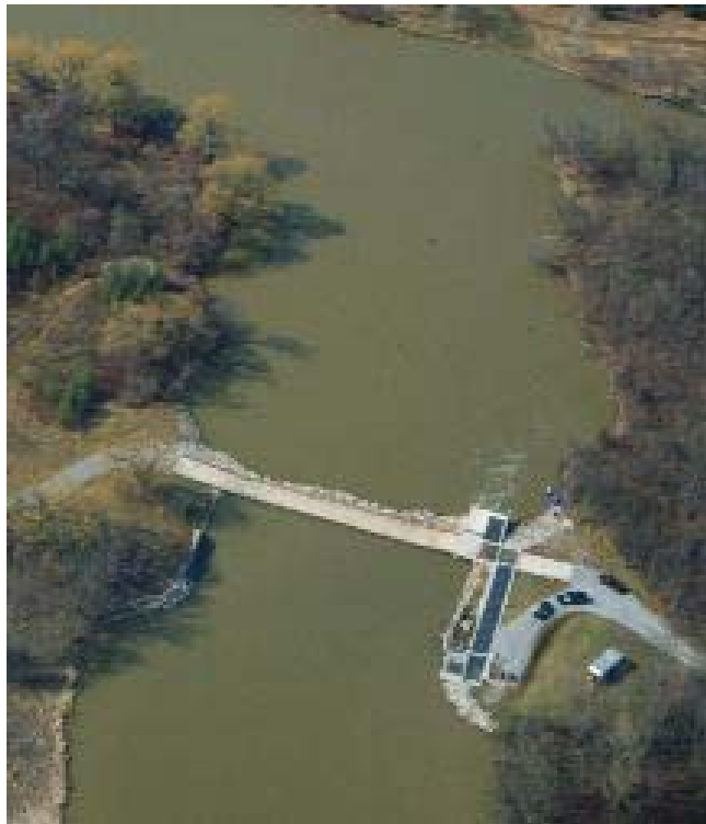
Figure 1.1. Aerial photographs of the Mannheim weir and two Denil fishways (top), and the Dunnville fishway (bottom), on the Grand River, Ontario.
